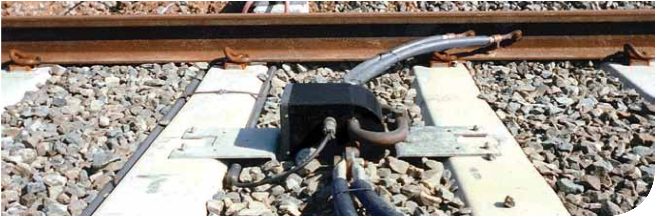
WEE-Z Impedance Bond installed at customer location
