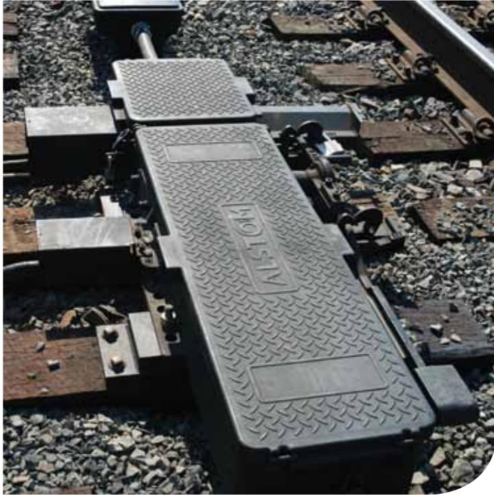
GM4000A™ Switch Machine installed at customer location
