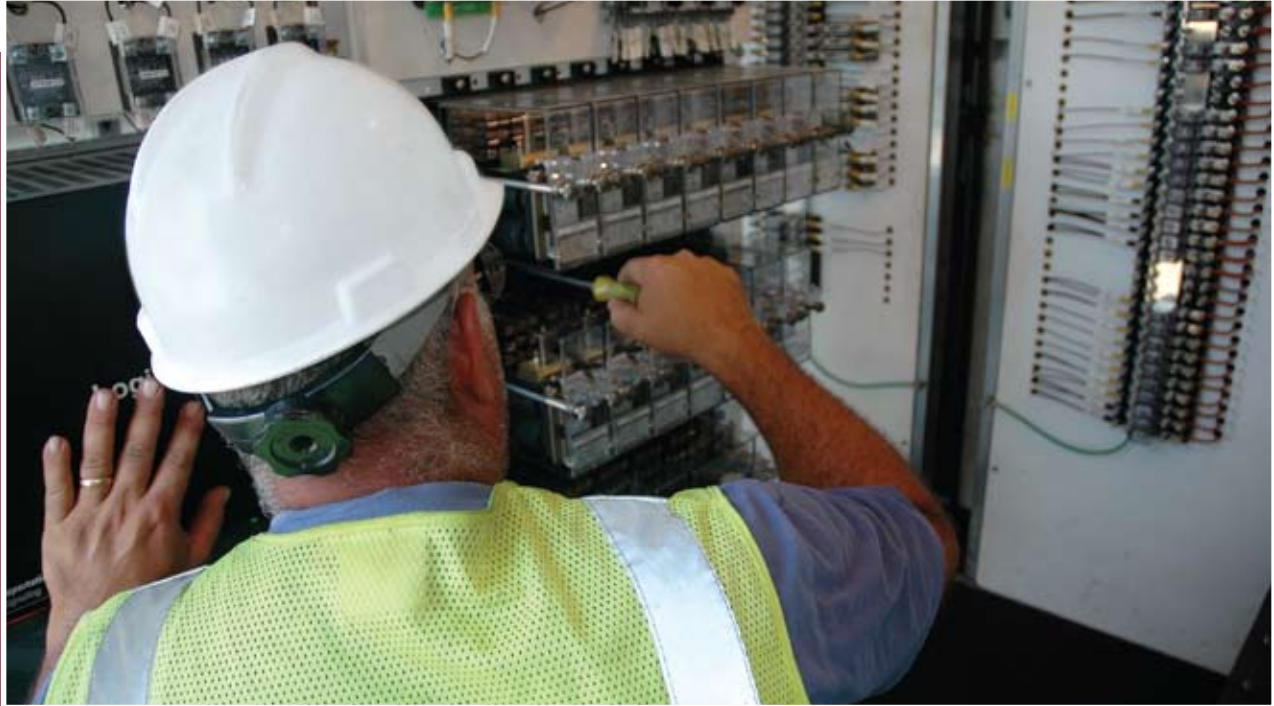
Relay Inspection at Customer Location
