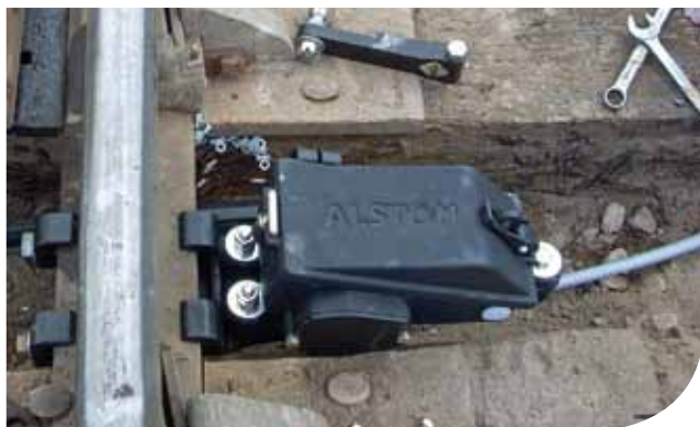
7R Switch Circuit Controller being installed at customer location
